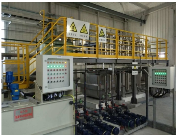
GEM System Installation
